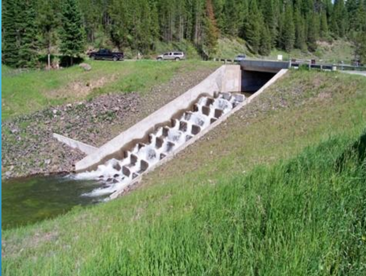
Dam with Baffled Spillway outside Bozeman, Montana
