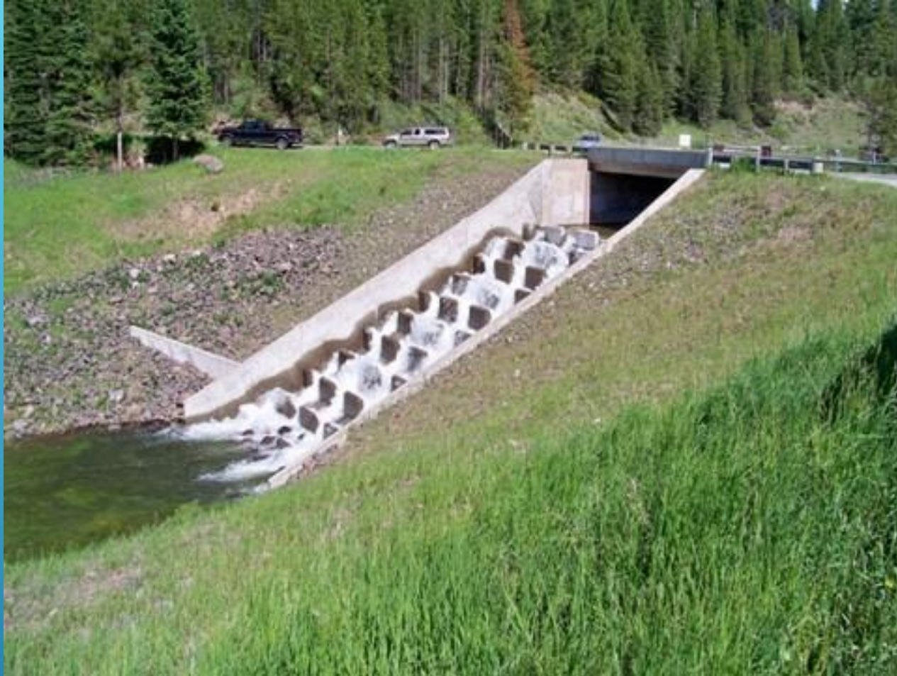
Dam with Baffled Spillway outside Bozeman, Montana
